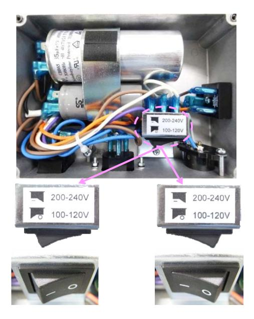
1-phase, 100-120V class power source 1-phase, 200-240V class power source Fig. 6 Changeover switch in the terminal box
